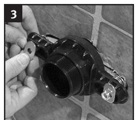
Install the uni-coupler with 3 spacer washers on each stud between the uni-coupler and spud flange. Then install the drain line test cap.
