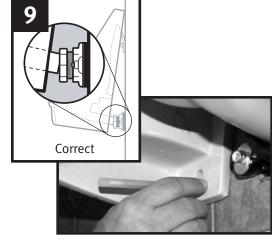
Re-hang and recheck bowl alignment with Drill holes for the lower anchor screws. the drain line. Mark anchor holes then remove the bowl.
