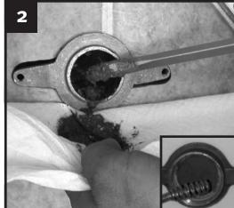
Scrape the drain line nipple to ensure there is no build-up. Then, auger the line to ensure there is no blockage.
