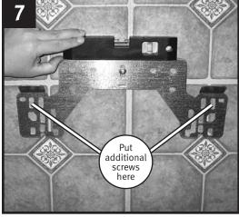
Level the bracket then drill two more holes on each side and install additional screws. If pre-existing bearing rods can be and adjust the bracket as needed. used, screws are not necessary.
