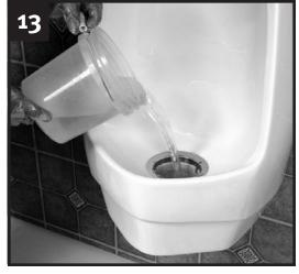
Perform water test to ensure good flow and verify there are no leaks.
