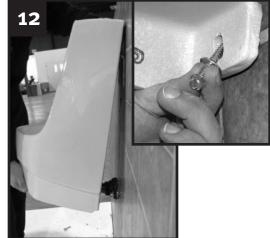
Hang the bowl, tighten uni-coupler fittings, and install anchor screws with washers.
