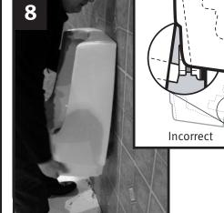
Hang the bowl on the bracket and check tail pipe alignment, then remove the bowl
