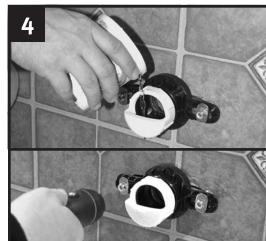
Slowly add water then check pitch/slope with flashlight. There should be no water present in the cap or nipple.
