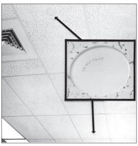
The Concealer® is designed for use where aesthetic appearance is important. Offices, hospitals, motels and restaurants are but a few of the applications where it can be used. It is available in different orifice sizes allowing the designer to optimize system performance, thereby achieving a most efficient installation.
