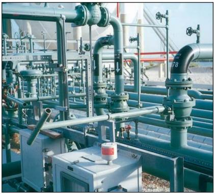
Velan *Memoryseal*<sup>™</sup> Ball Valves can be equipped with electric, pneumatic, hydraulic or gear actuators.
