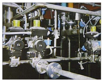
**Photos on page 26**: Split-Body ball valves installed in a chemical plant in Ohio.
