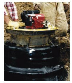
WrapidSeal™ - positive external seal; vacuum tests to 11" Hg.
