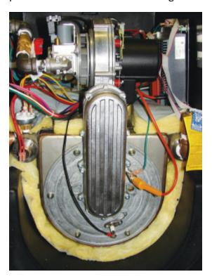
individual stainless steel water circuits are baffled to direct the flow which maximize the heat
