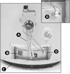
$\hbox{A. Industry standard thermocouple}\\$
