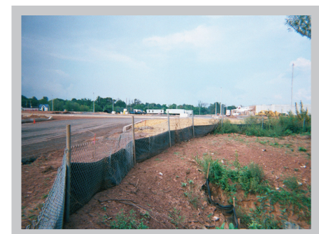
Super Silt Fence - Wire Backing
