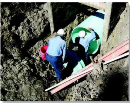
Each male end shall be beveled to facilitate joining and referencing marked for proper insertion depth. Diamond furnished lubricant is to be used in the joining process.
