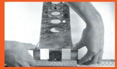
Attach bracket to t-bar ceiling grid.
