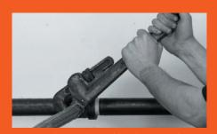
Connect FlexHead sprinkler drop to submain.
