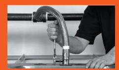
Secure FlexHead sprinkler drop to bracket.
