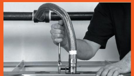
Secure FlexHead sprinkler drop to bracket.
