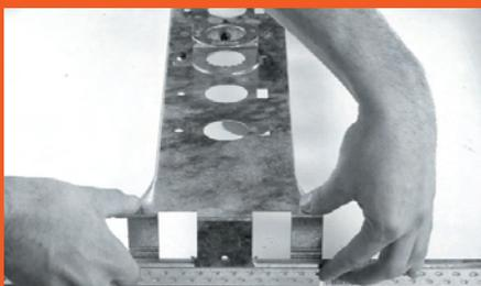
Attach bracket to t-bar ceiling grid.
