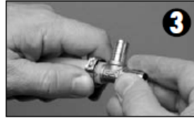
3 Push the PEX tubing onto the fitting against the fitting shoulder.
